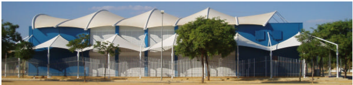
Figure 4: Extensión of Pío XII school in Bollullos de la Mitación, Seville (J.C. Gómez de Cózar, 2004). Roof composed of a combination of opaque and transparent membranes framed by tubular section arches. Membranes give lightness and help for quickly assembling. They are easily replaceable.
