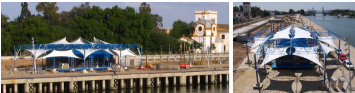
Figure 2: Project of travelles' reception module. Seville's Port (J.C. Gómez de Cózar, 2005). Surrounding of existing metallic lattice window by means of four different geometries with all the free edges cloths. Besides to contribute to reduce the tempereature in the inferior cockpit, it is constituted like a landmark in the city.
