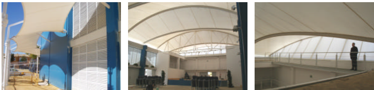
Figure 5: Multiuses Centre in Pilas, Sevilla (J.C. Gómez de Cózar, 2004-07). Building solved by quickly assembled proceedings. Membranes play a double role: MAIN (the roof. It was built in one week), SECONDARY (perimetral gallery. It defines a circulation space around building and gives shade to façade).
