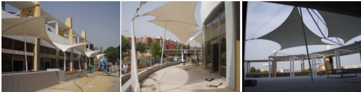
Figure 3: Project of comercial galleries and shadow areas for the shopping centre Zona Este in Seville (J.C. Gómez de Cózar, 2006). Arches and free endings are brought together in the galleries. All elements give shade and are used as advertisement.
