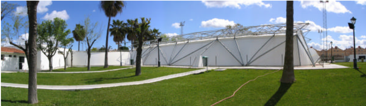
Figure 1: Covered and air-conditioned swimming pool in Gines (Sevilla). Unfolded mesh composed of two layers of rhombuses and scissors. A continuous and tautened textile membrane hangs from it.
